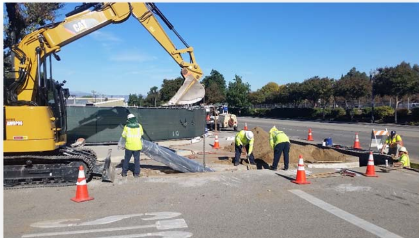
Service Installation – Hotel Luxen
