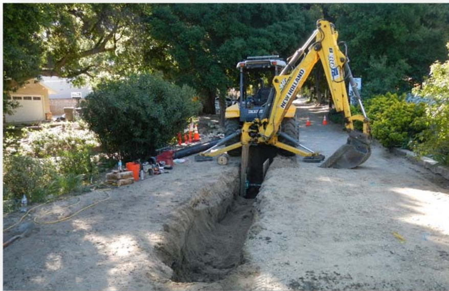
Mainline Replacement – Cross St.
