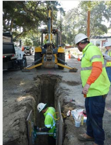
Pipeline Replacement – Cross St.
