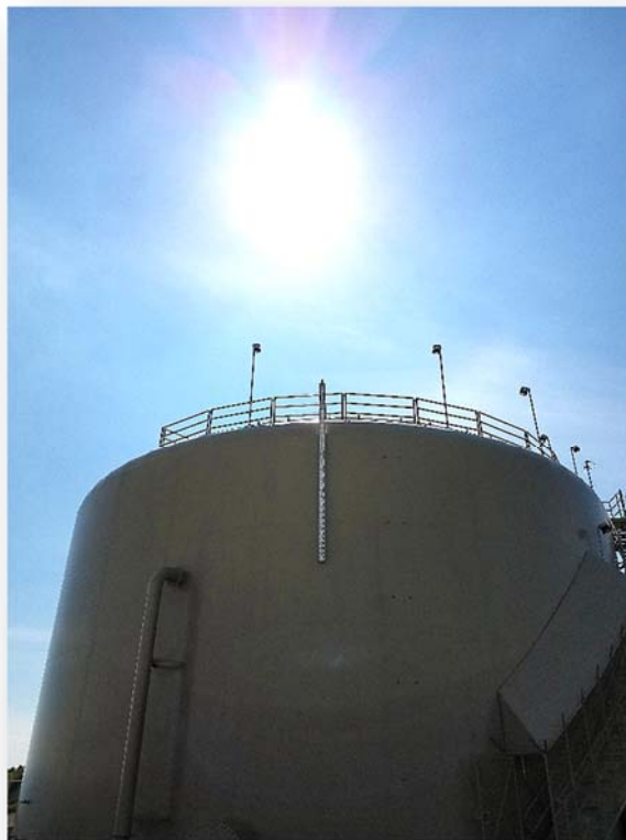
New Castaic Tank No. 3
