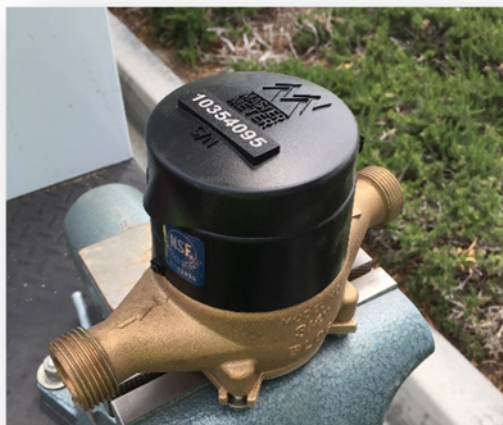
Meter Replacement – Master Meter
