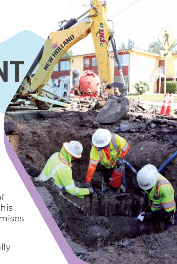
MAINLINE REPAIRS IN NEWHALL
