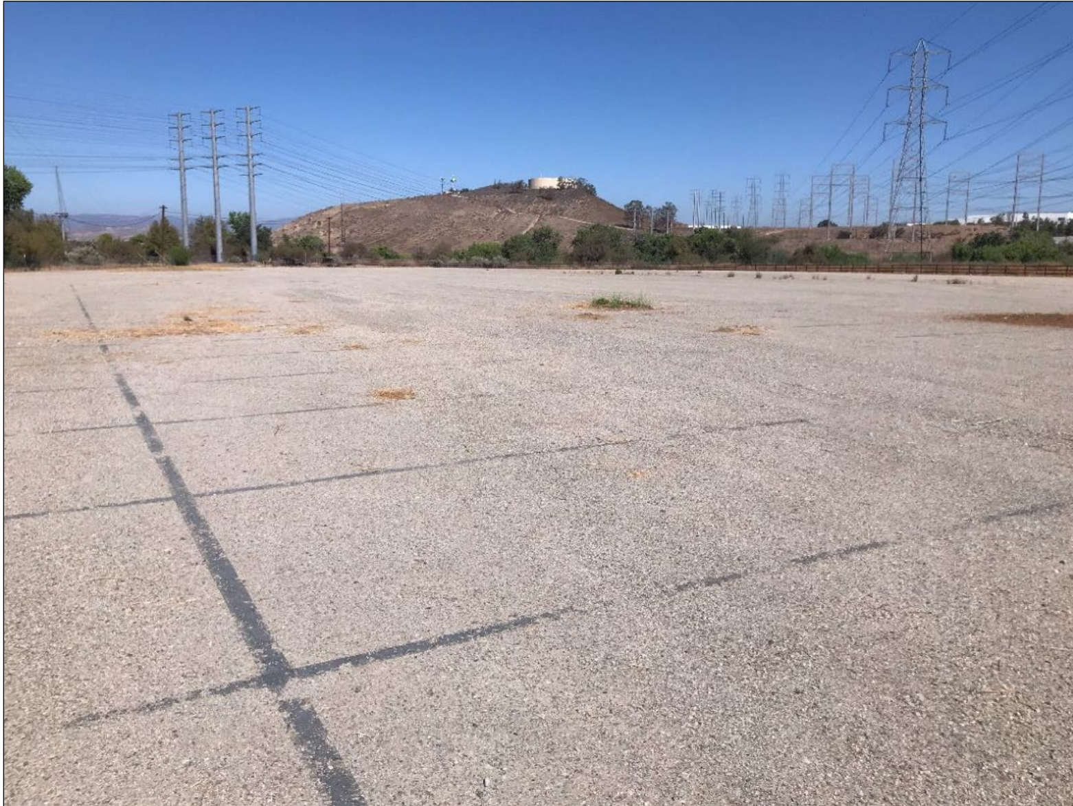
Figure 2-13: Backcountry Pump Station Site, Facing Northwest
