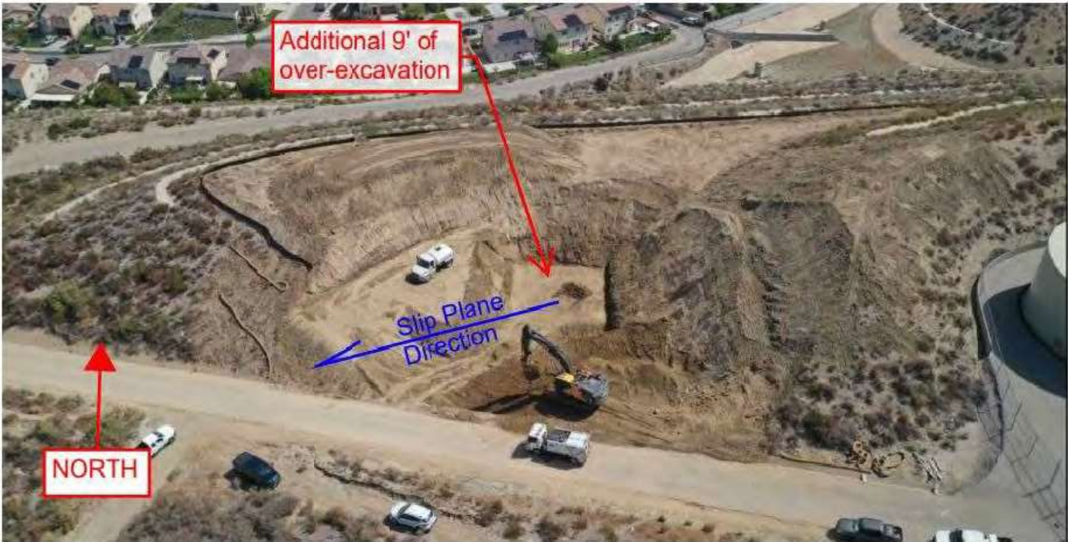
Photo of Over-excavation and Backfill on 5/14/21
