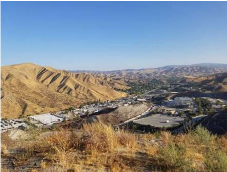
Photo 4: Project Site Overview (View NE)
