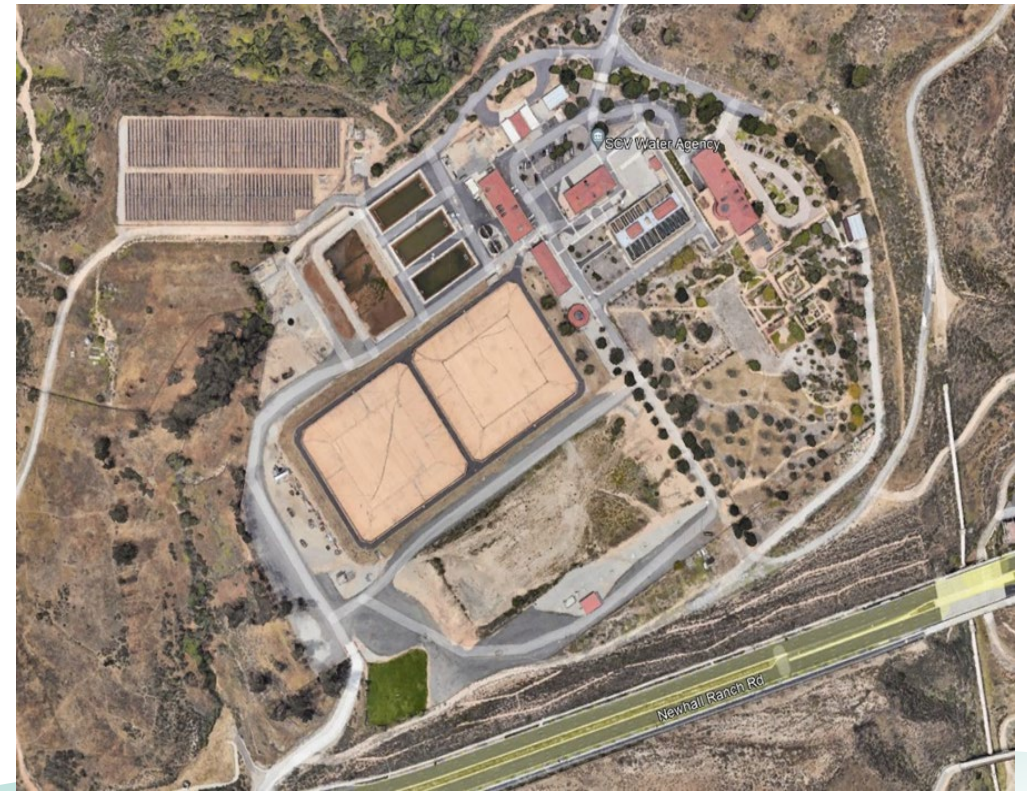
Rio Vista Water Treatment Plant – 66 MGD
