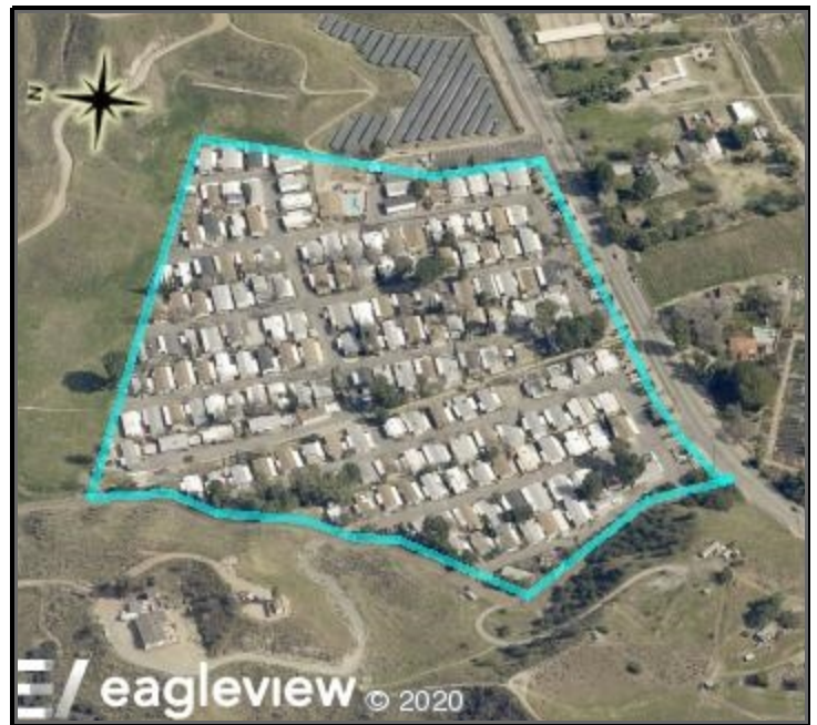
View Looking East
