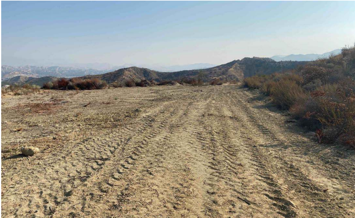
Photograph 1. View of Modified Project graded pad site, taken from southwestern portion of site facing northeast.
