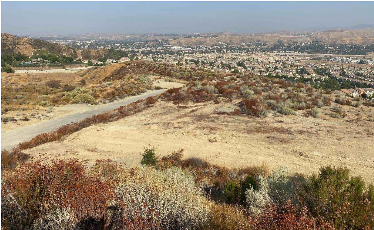
Photograph 2. View of Modified Project graded pad site in foreground, access road and pipeline corridor and Original Project graded pad site in mid-ground, and Fair Oaks residential community in background. Photo taken from existing berm directly south of Modified Project site, facing northwest.
