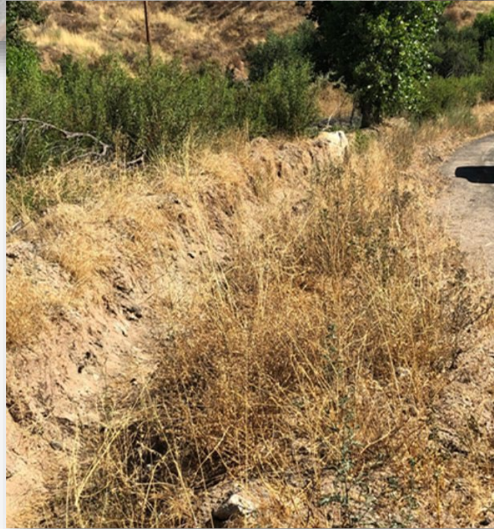
Culvert between Bouquet Creek and Bouquet Canyon Road
