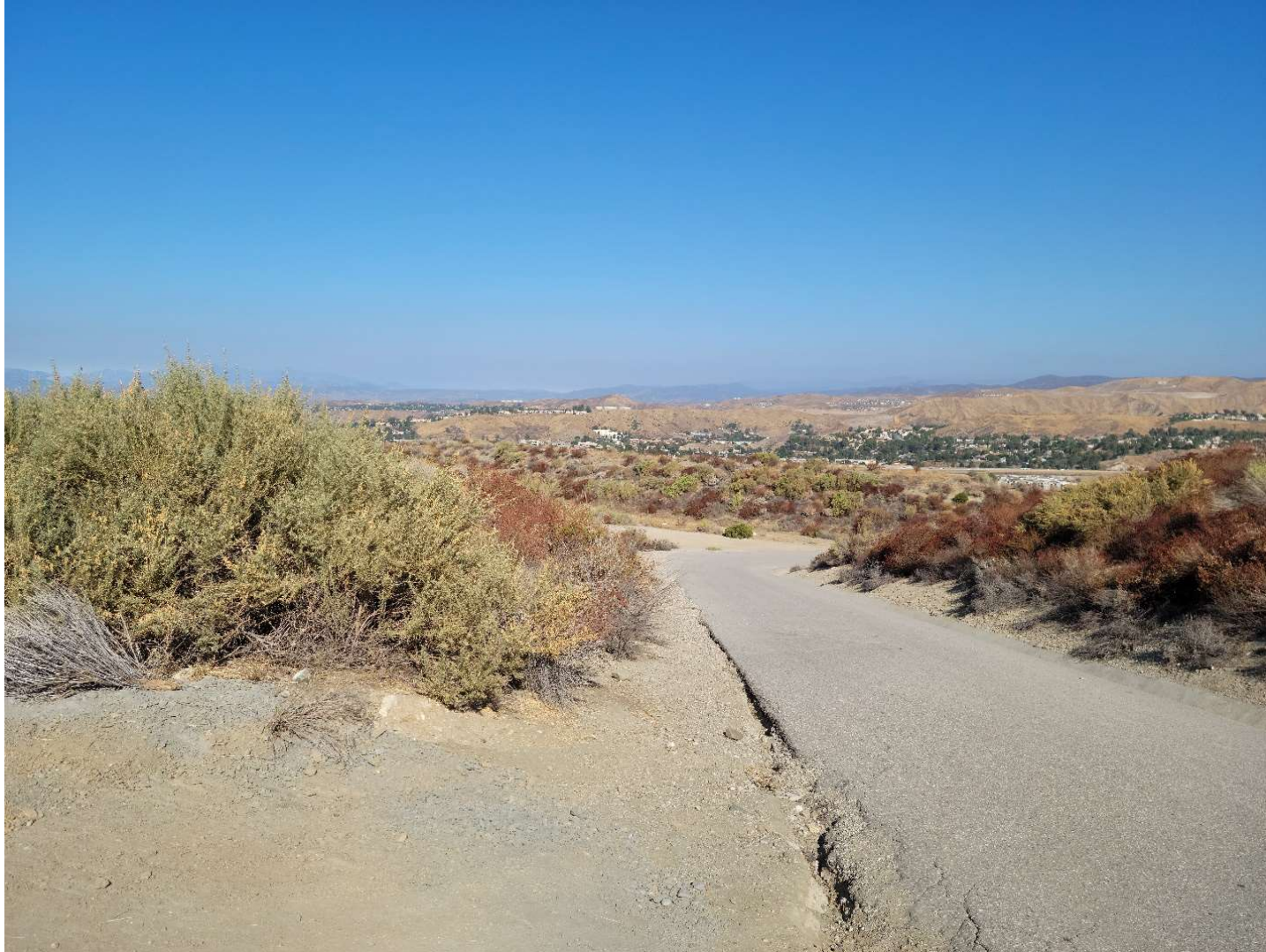
Figure 6 Overview of Pipeline Extension Area, Facing North
