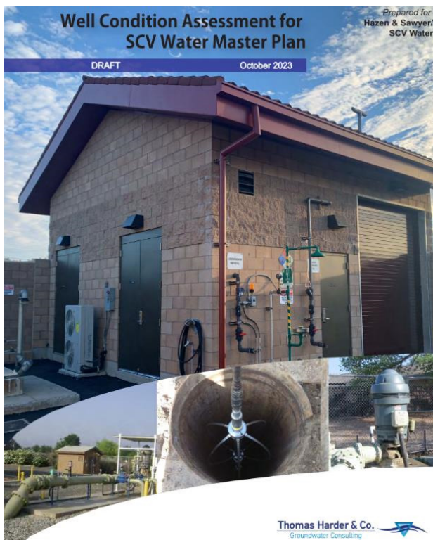
Well Condition Assessment
