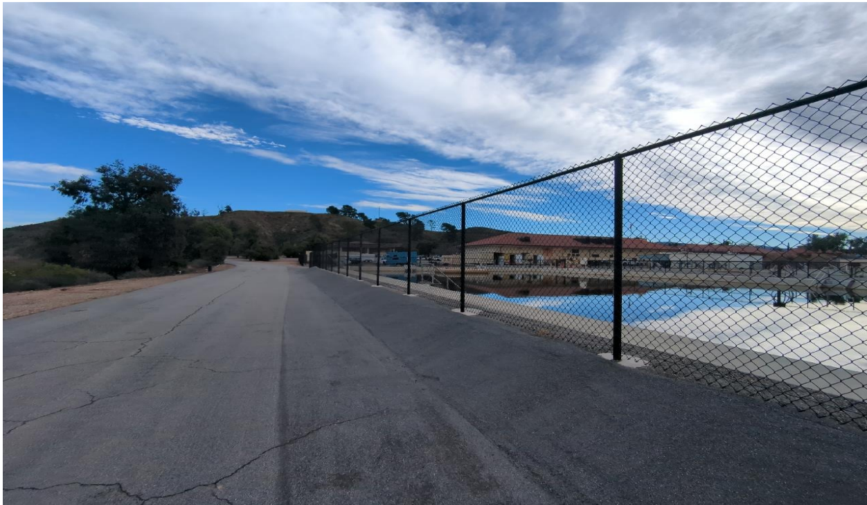
Photograph 14. View of existing water treatment facility associated with the RWTP, facing east.
