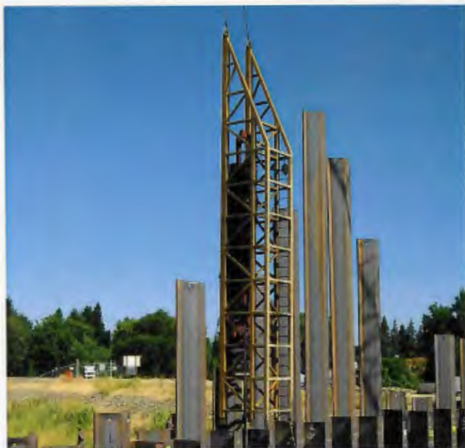
Driving steel sheet piles with an impact hammer
