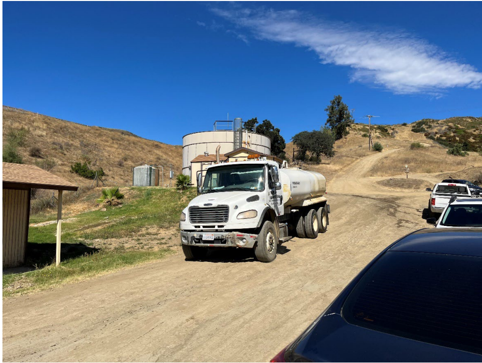
Overview of On-Site Tank Location
