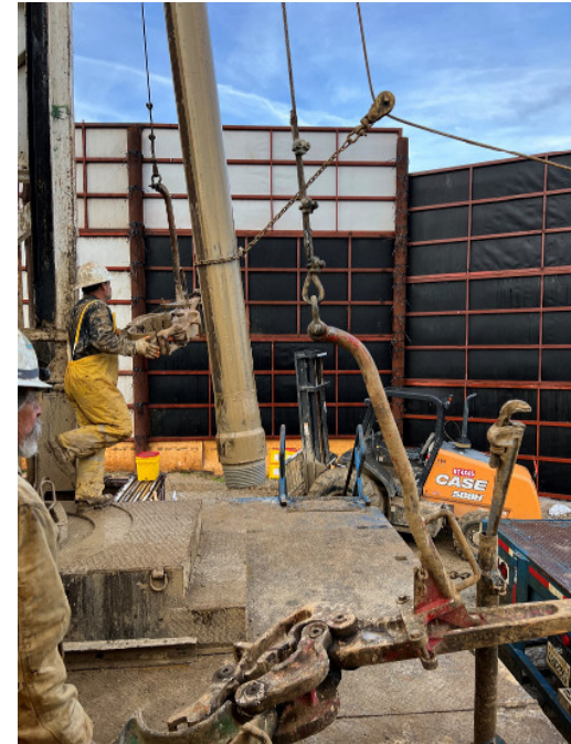
Pilot Hole Drilling
