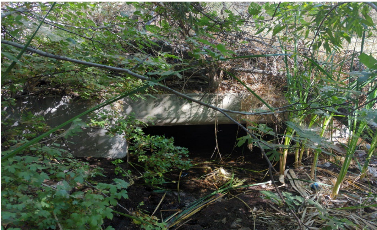
Photograph 26. Photo Point 26. View of the Intermittent Drainage 1 culvert outlet that transports flows underneath SR-14 and into the APE, facing north. Note large amount of sediment deposition and riparian vegetation (August 4, 2023).
