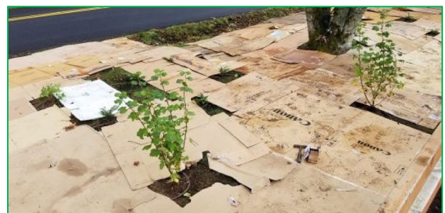
2 Accelerated Planting Sheet Mulching: Sheet mulch, cut holes in the cardboard, and plant trees and shrubs at any point in the sheet mulching process.
