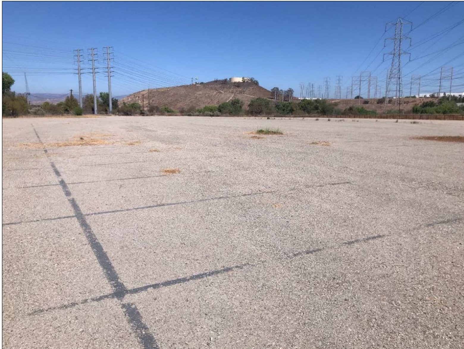
Figure 2-13: Backcountry Pump Station Site, Facing Northwest
