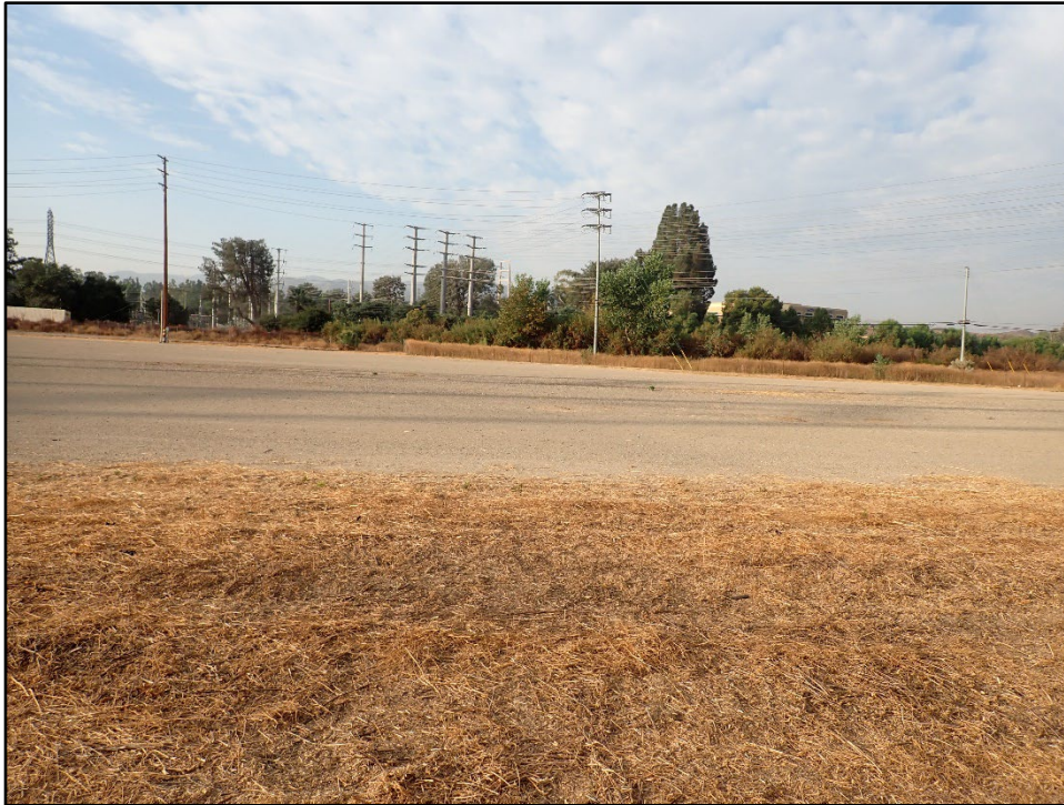
Figure 9. Project overview, view facing southwest.
