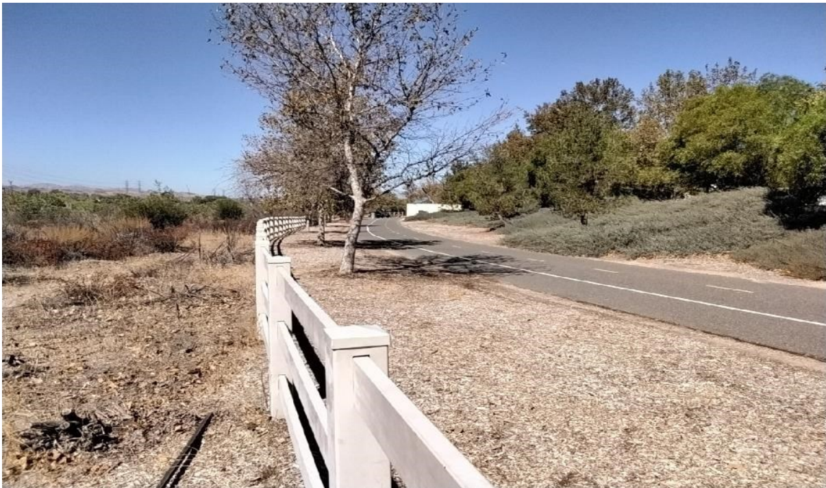
Photograph 24. Photo Point 24. View of the proposed pipeline improvements along the Santa Clara River Trail, facing west. Note the existing Well S8 facility in the background (August 30, 2022).
