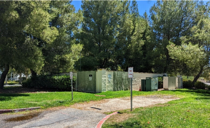
Photograph 3. Existing S6 well enclosure, view from the west.
