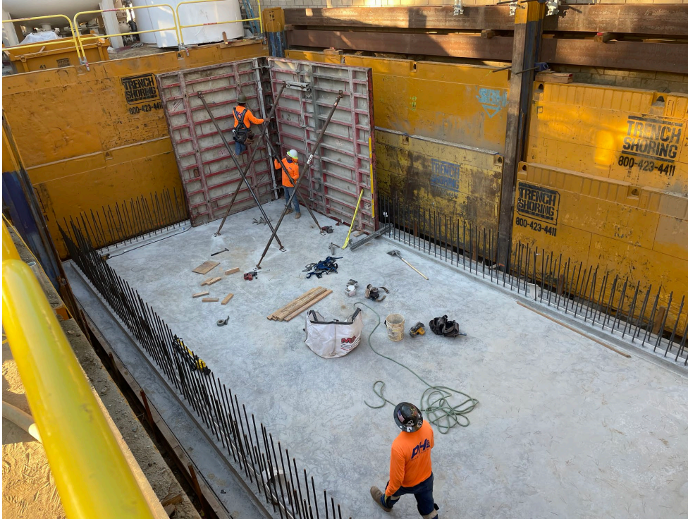
Installing formwork for underground backwash tank
