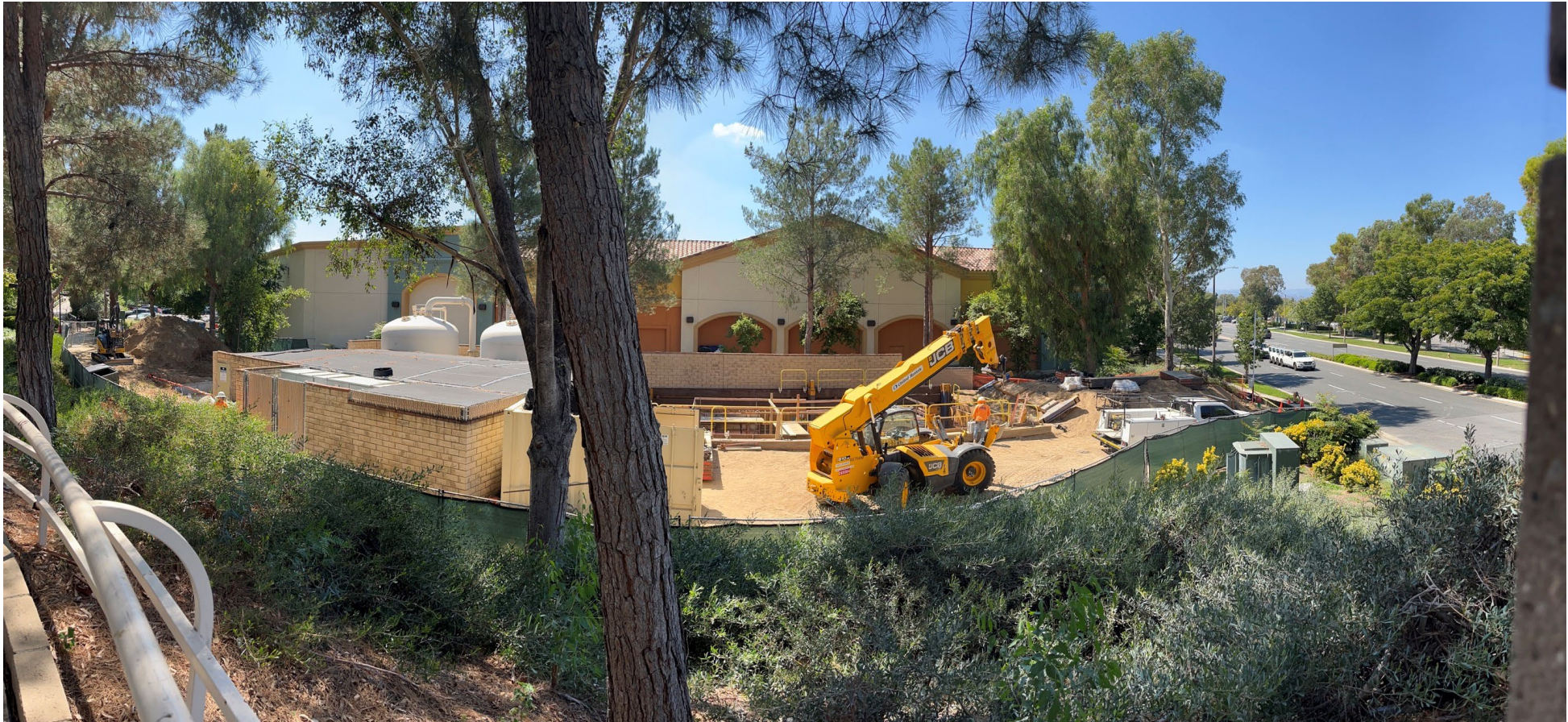
Overall site (September 18, 2023)
