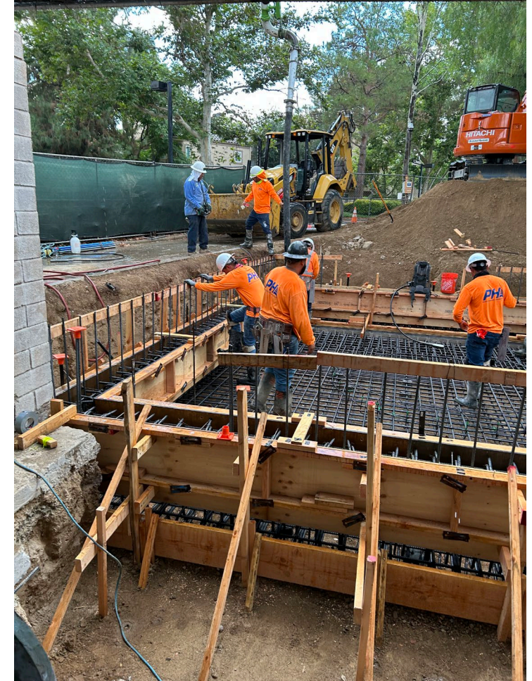
Installing formwork for Chemical Building Foundation
