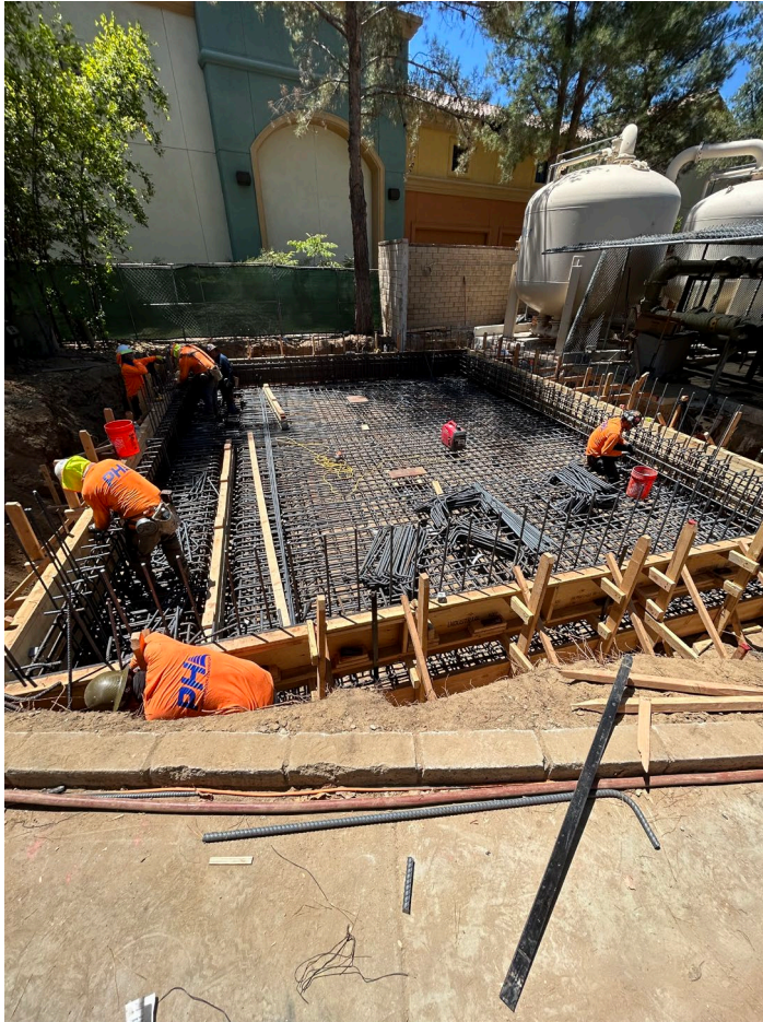
Installing formwork for Chemical Building Foundation
